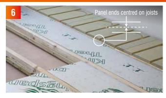
To allow for the wood's natural movement in service, the boards should be laid so, that a gap of at least 10mm is left between the boards and the walls and between the rooms. The end returns should be glued and screwed in the same way as the straight boards.
