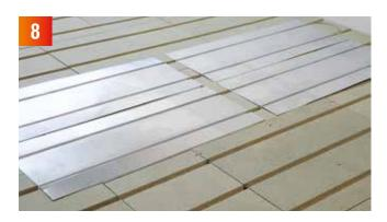
The heat transfer plates are installed by pressing them to the straight sections of ProFloor boards. The distance between the heat transfer plates has to be 10-100mm. There is no need to attach the heat transfer plates to the base.
