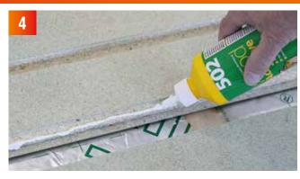
The boards should always be glued to each other at the tongue and the groove. The boards can also be glued to the base to avoid possible creaking. The glue should be an appropriate PVA wood glue. Application of the glue should be done carefully ensuring that there is a continuous seam of adhesive along the entire length of the tongue and groove. Note however that excessive use of glue might lead to gaps between the boards.
