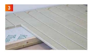
It is recommended to start installation at the furthest place from the water manifold to enable easy installation of the transfer pipes between the piping and the manifold.
