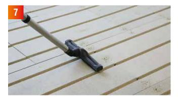
Before installing the heat transfer plates, the floor and the piping grooves should be cleaned of sawdust and other dirt.
