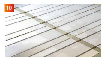
70-90% of the floor area should be covered by the heat transfer plates. The floor should be cleaned once more before the installation of the pipework.
