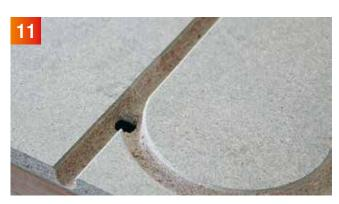
The inlets are milled before installation of the boards or directly to the floor surface.
