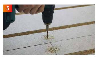
ProFloor boards should be screwed to the base with screws suitable for screwing wood. The screws should be countersunk screws  $50-75 \,\mathrm{mm}$  in length. The screws are attached to the middle and the edges of the boards  $300-450 \,\mathrm{mm}$  apart.
