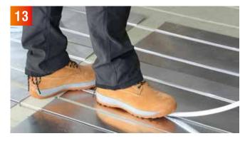
Install the heating pipes into the grooves of the heat transfer plates. Make sure, that the pipe is fully embedded to the groove to avoid it carrying load under the final floor surface. To ensure the pipe sits flat into the groove, lay the coil of the pipe flat to the floor
