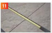
Use a small piece of the underfloor heating pipework to place in between the groove joining two boards. This will help to keep the floor in place.
