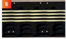
Start to roll the pipe into the Overlay End Support, utilis ing the selfretaining pipe clips, and continue to push the pipework into the connecting pipe runs until you reach the other end of the room.
