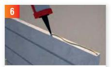
Work your way back up the room, staggering the panels as you go. Ensure you apply the 3mm bead of Overlay glue to all edges.
